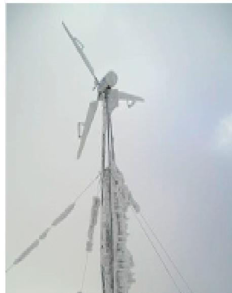
**Fig. 1.** *Condition of the wind-driven power plant after a snow storm*
