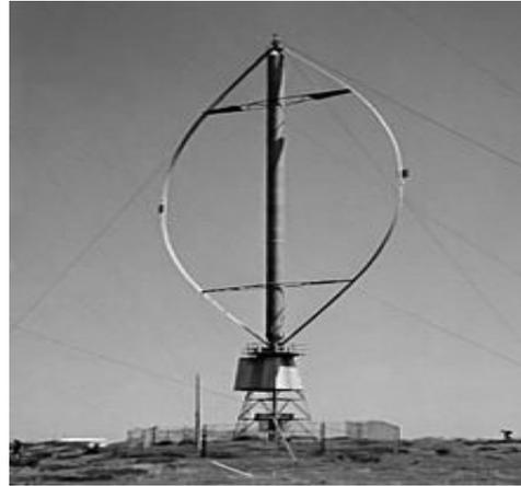
*Fig. 2. Darrieus wind-power unit of troposkino system*
