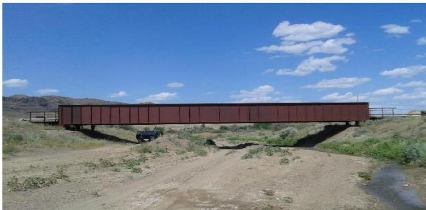
Fig. 1. General view of the beam superstructure of a metal bridge and a railway track laid on wooden beams with a ride on the bottom
