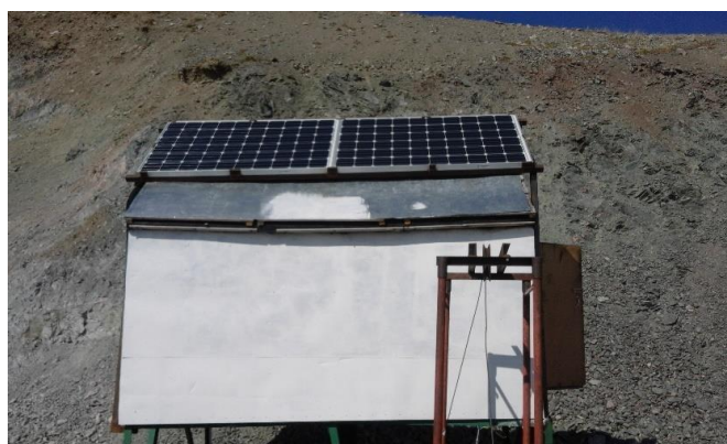
Figure 4. Special room with solar panels installed in its roof.
