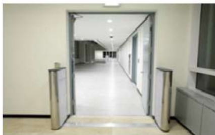
(4) A fixed-type RFID reader checks all records taken in and out of the storage
