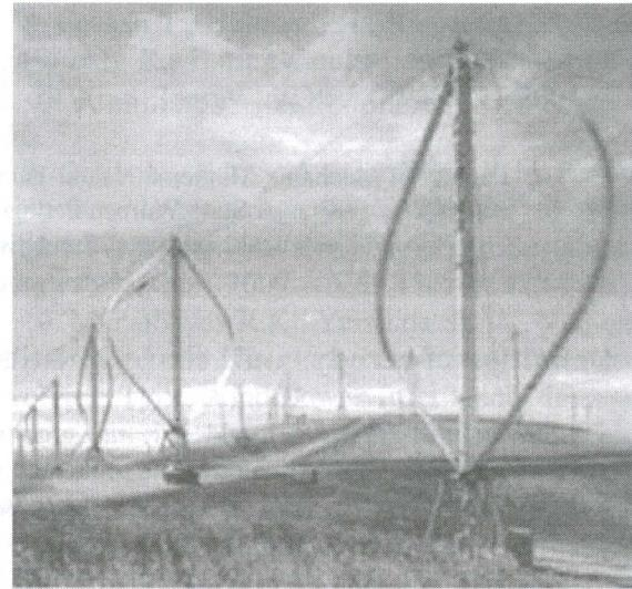
**Figure 1** – Wind turbine with the turbine to Darrieus of system troposcino
