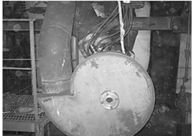
**Fig. 4.** General view of the vortex PFS with a scroll for the BKZ-420 boiler at the Almaty CHP-2.
